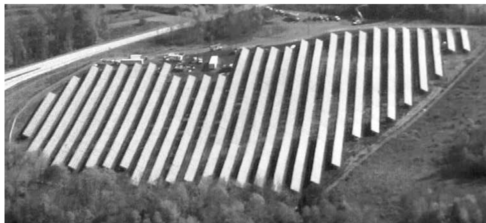
Larger solar projects, like this one in Williamstown, are cropping up more frequently in Vermont. As they proliferate, and as proposals for new ones become much larger than this, some members of the public have grown concerned about land use. The draft PSB net metering rules are one place where this concern is taken into consideration.
