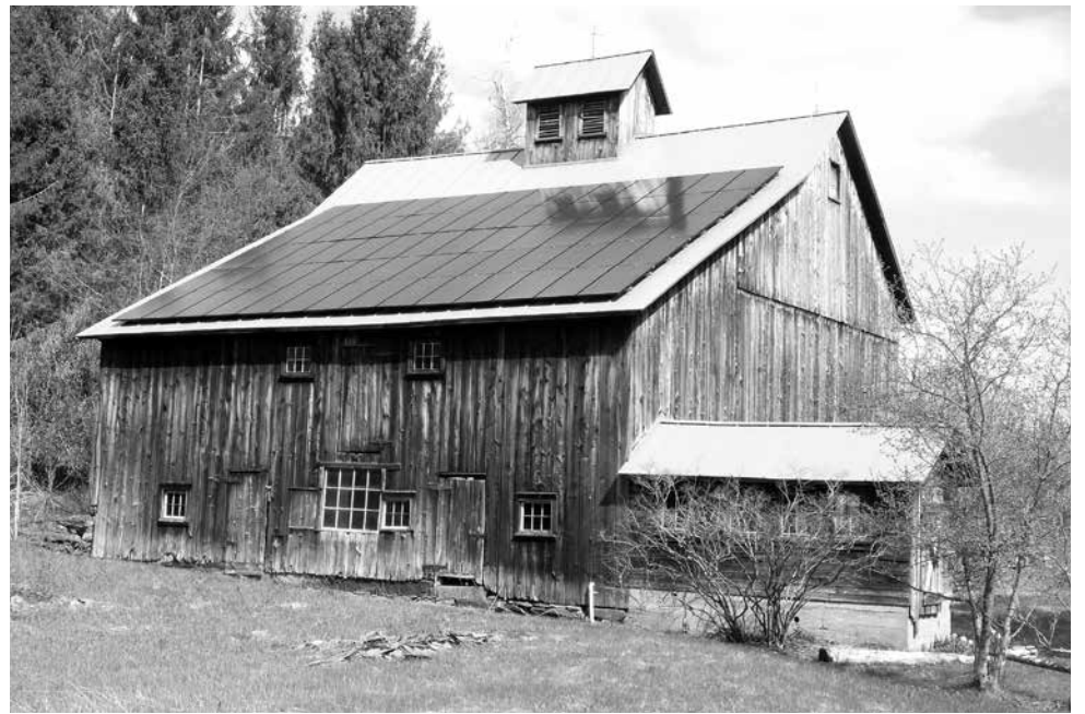
Home-sized solar net metering systems typically generate power from panels on the roofs of houses – or, in this case, somewhere in Vermont – a barn, or outbuilding. Some are placed on racks built upon the ground.
